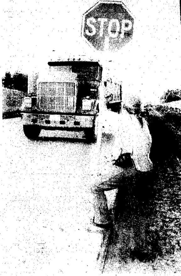
Linda Johnson stops traffic on Highway 15. The construction project will be completed within three weeks.
